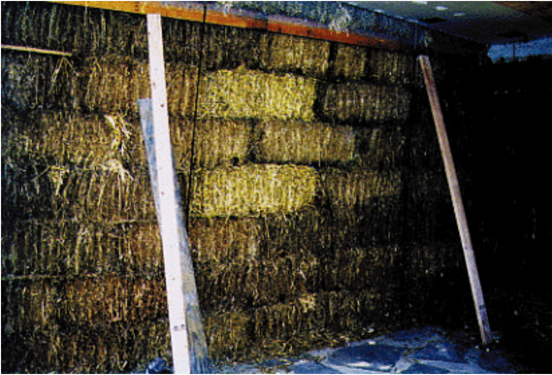
Figure 5, showing completed wall with four new bales inserted. When two-by-fours were removed, the wall settled back to its original configuration with no obvious negative consequences.
