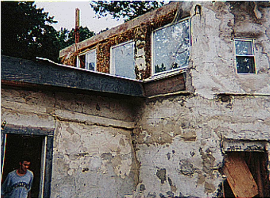
Figure 2: The clearstory windows from the opposite direction. Wooden frames held the window in the walls of straw and wooden beams.
