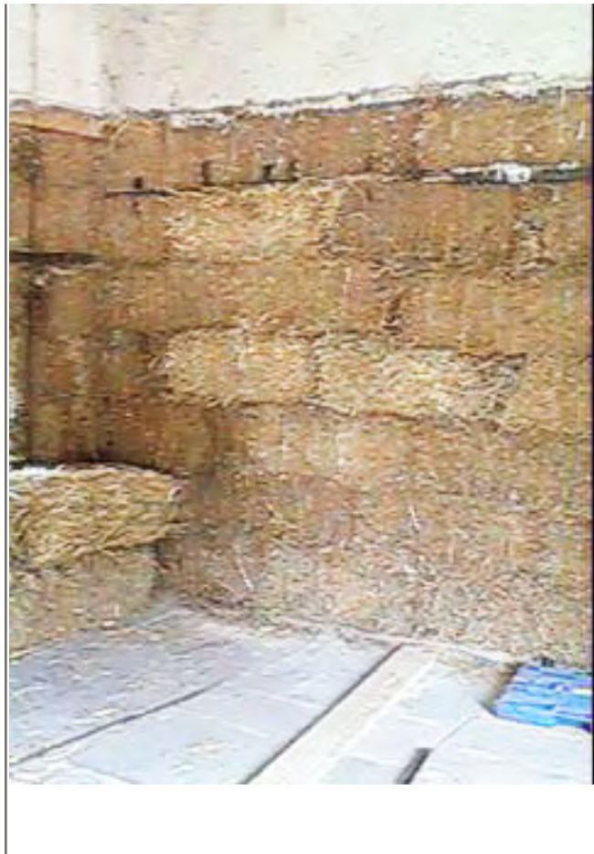
Figures 6 and 7, showing hole in load-bearing wall after removal of five bales, and completed wall with new bales inserted.
