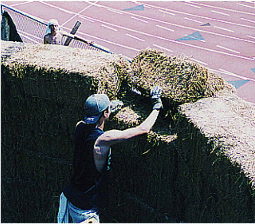
Figure 5a: A Straw Bale worker removes the very first bale.
