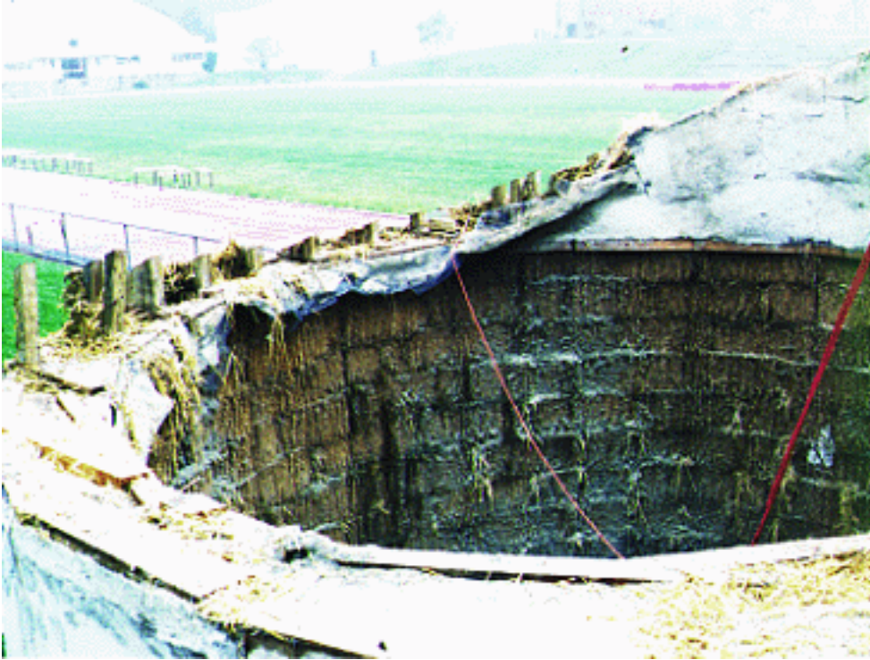
Figure 3: The bond beam which encompassed the top of the circular wall.
