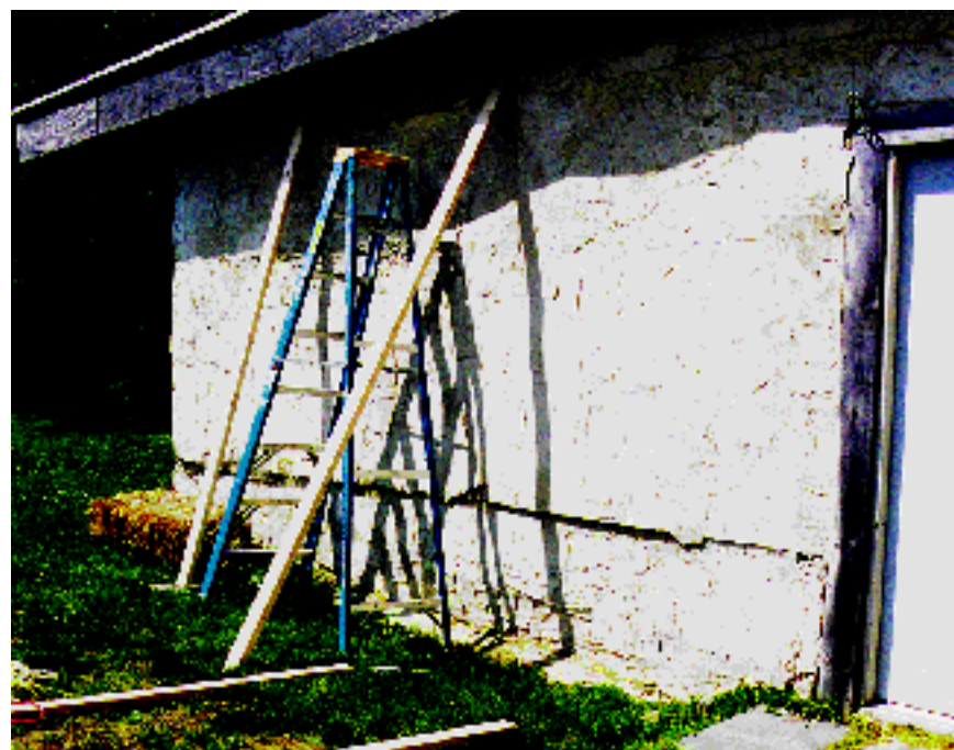
Figure 2, showing non-load-bearing wall outside stucco surface prior to in-situ bale replacement.
