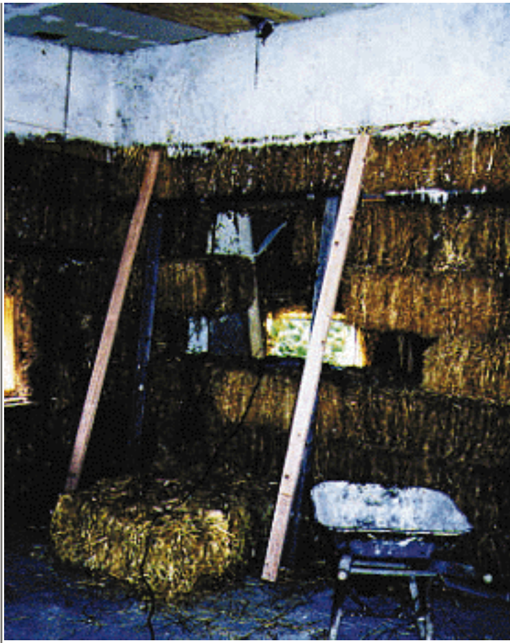
Figures 6 and 7, showing hole in load-bearing wall after removal of five bales, and completed wall with new bales inserted.
