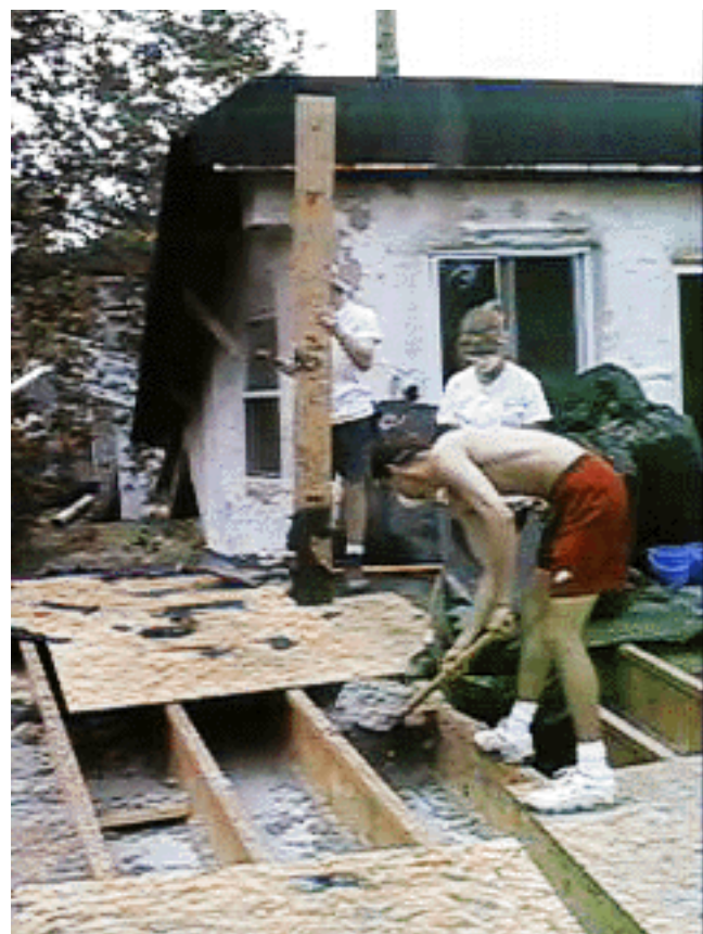
Figure 2. The insulation is shoveled into plastic trash bags.
