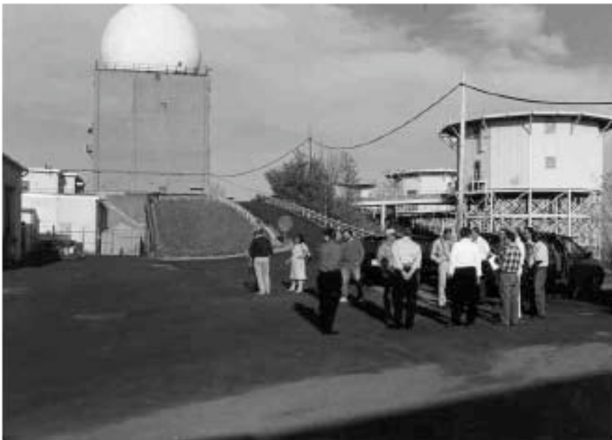
• Figure 4 - Former NIKE Control Area
